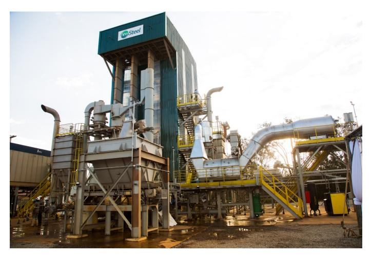
Pilot plant will have the capacity to concentrate 30 tons per hour of dry ore, using magnetic separation technology, made using rare earth magnets
