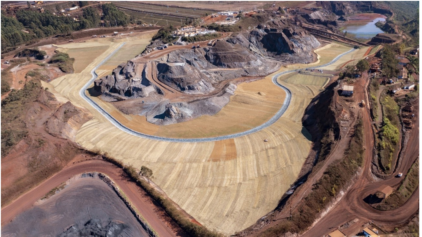
The Fernandinho Dam, in Nova Lima (MG), was one of the de-characterized structures.
