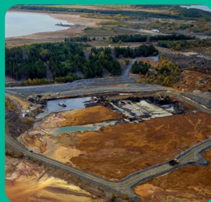
A tailings project area.
