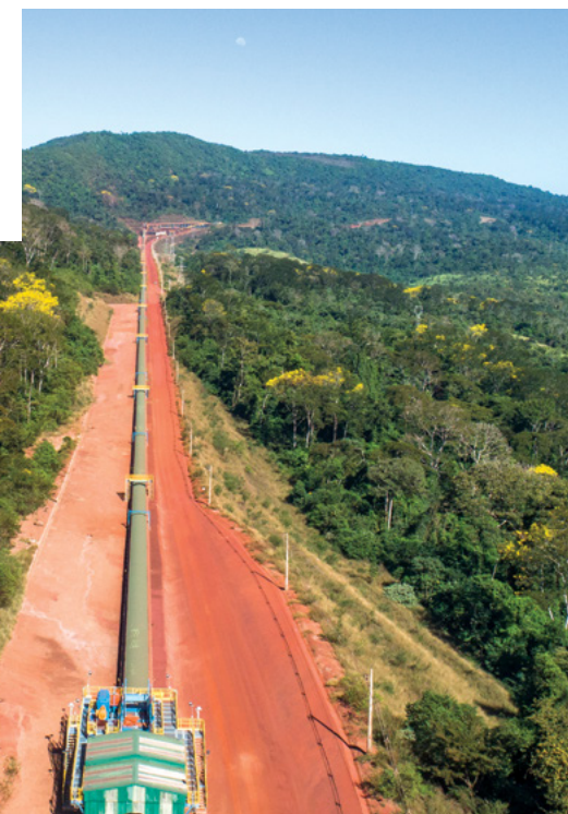
TCLD (in Portuguese) Belt System - Long Distance Belt Conveyor at the Eliezer Batista Complex in Canaã dos Carajás (PA, Brazil) Photo: Ricardo Teles
