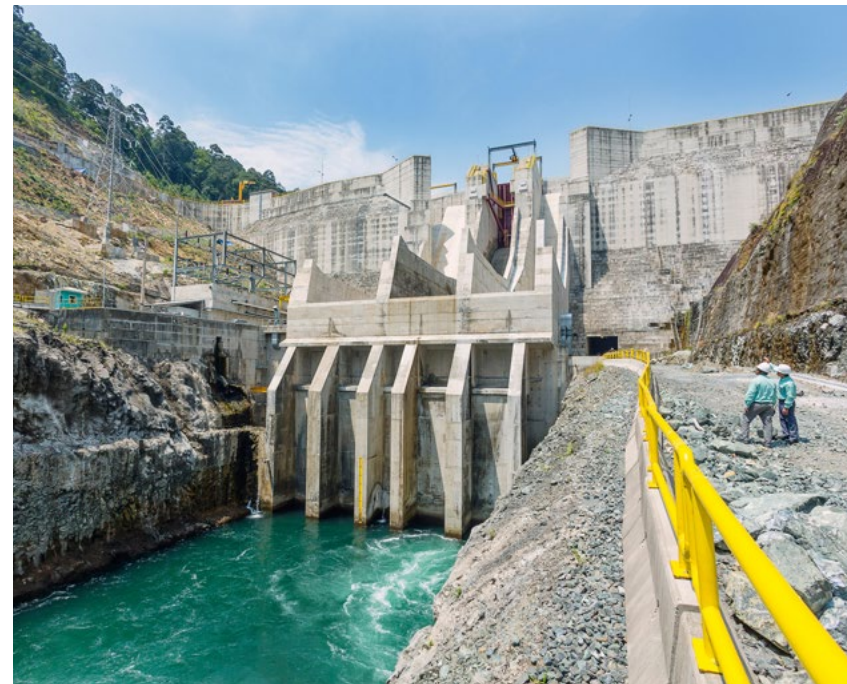
Karebbe hydroelectric plant, Indonesia
