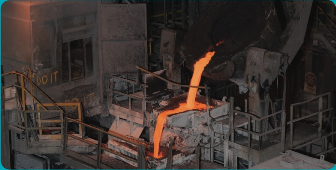
The automated anode casting section of the Smelter fills molds with molten Bessemer matte from the converters.
