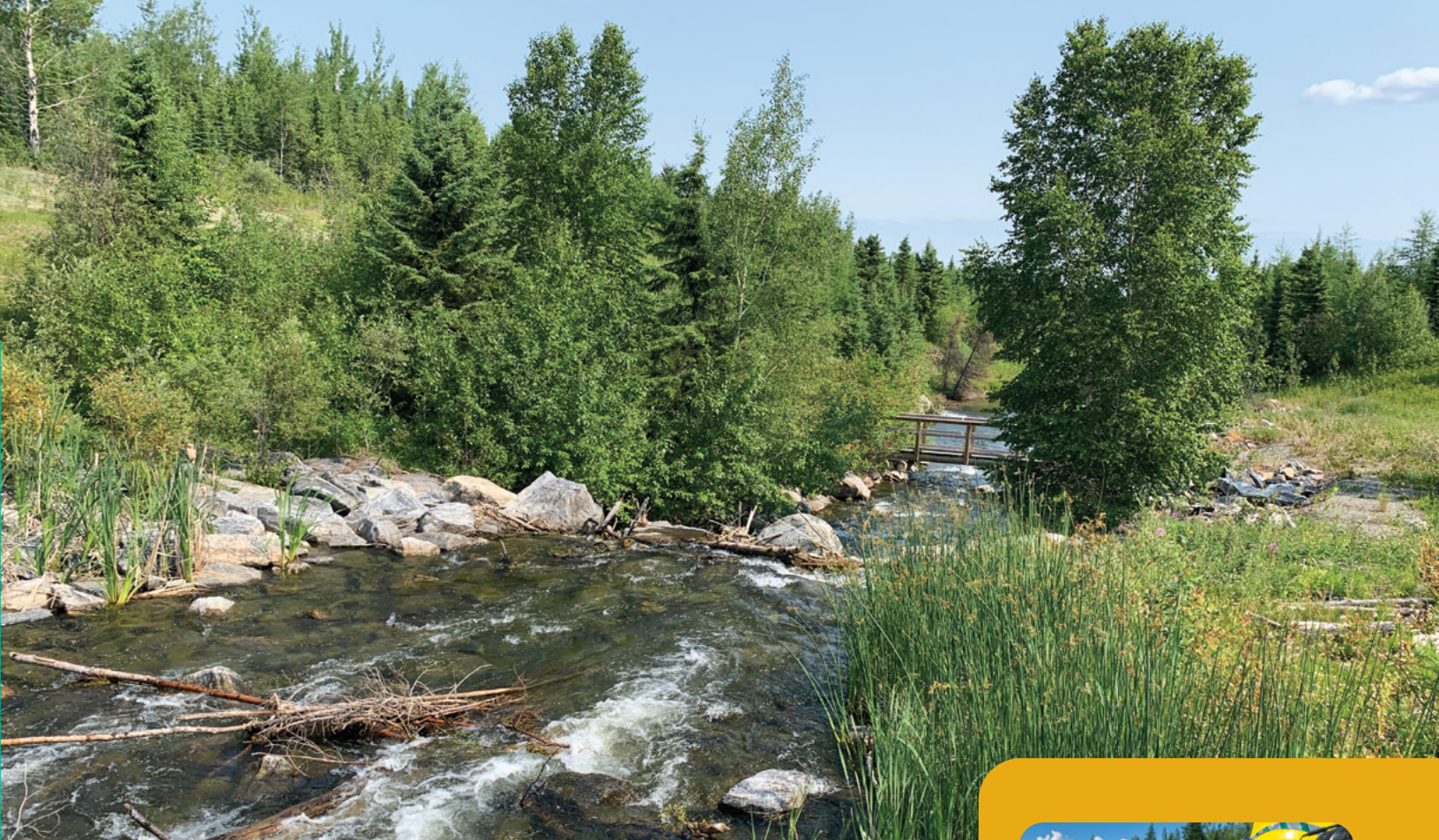
The fish barrier as seen at the weir final discharge point.
