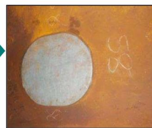
GEOTEXTILE INVOLVING ALL THE LID
