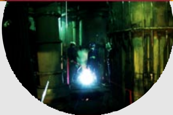
Pekerjaan pembongkaran atap Tanur Listrik No.3 (bawah). Demolition work on the roof of Electric Furnace No. 3 (below).
