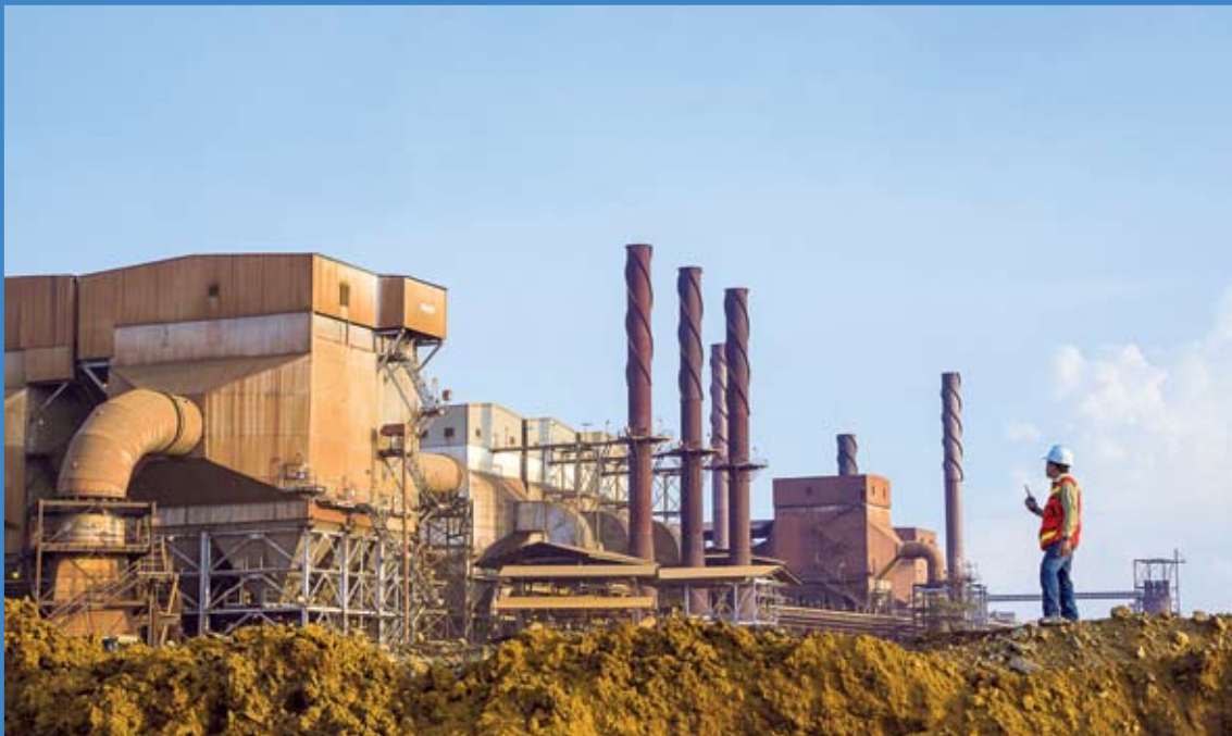
Pabrik PT Vale Indonesia Tbk PT Vale Indonesia Tbk plant
