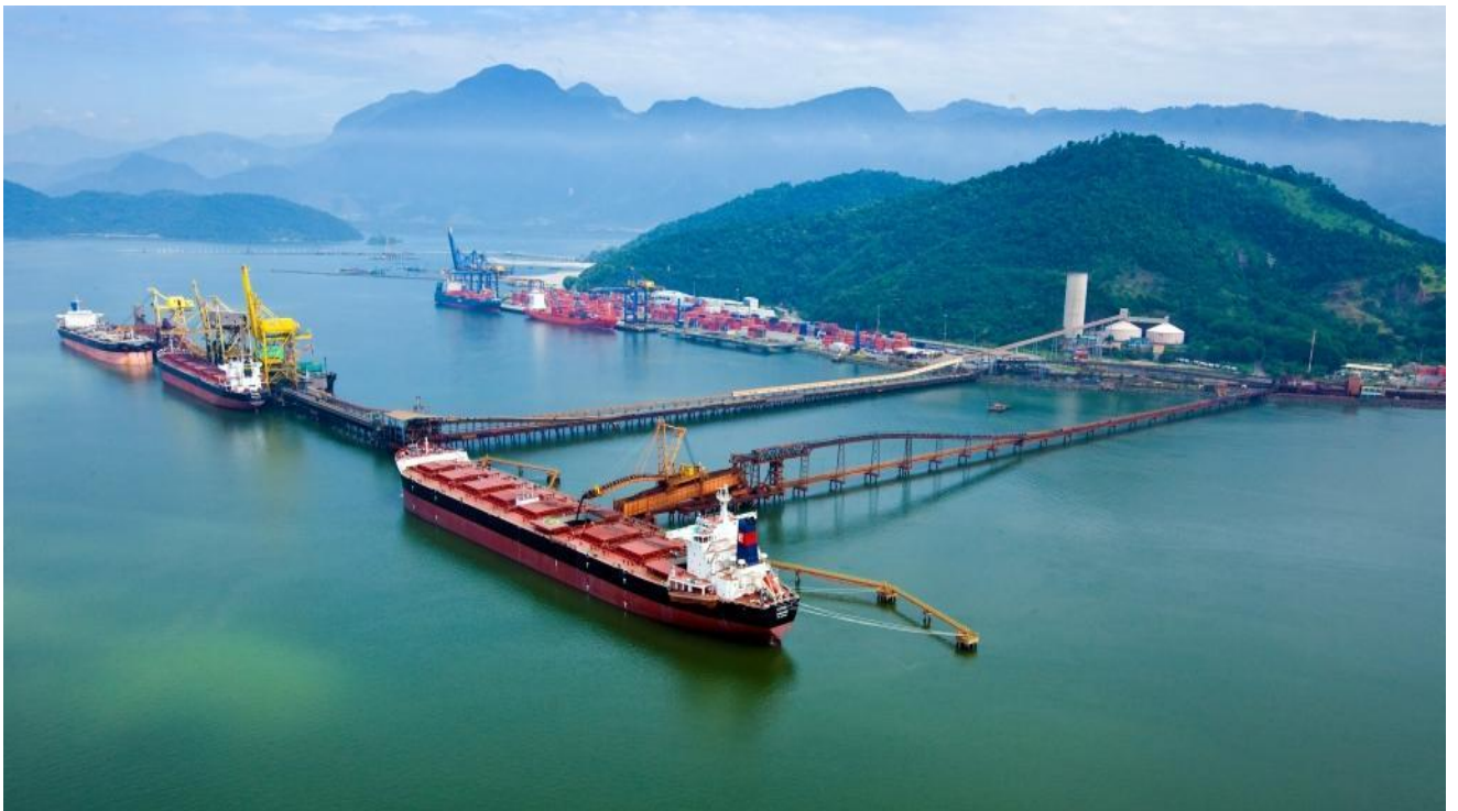
Figure 1 - Panoramic view, in the foreground, of the CPBS Terminal
